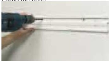
Oblong perforations for quick fitting and easy adjustment of the base
