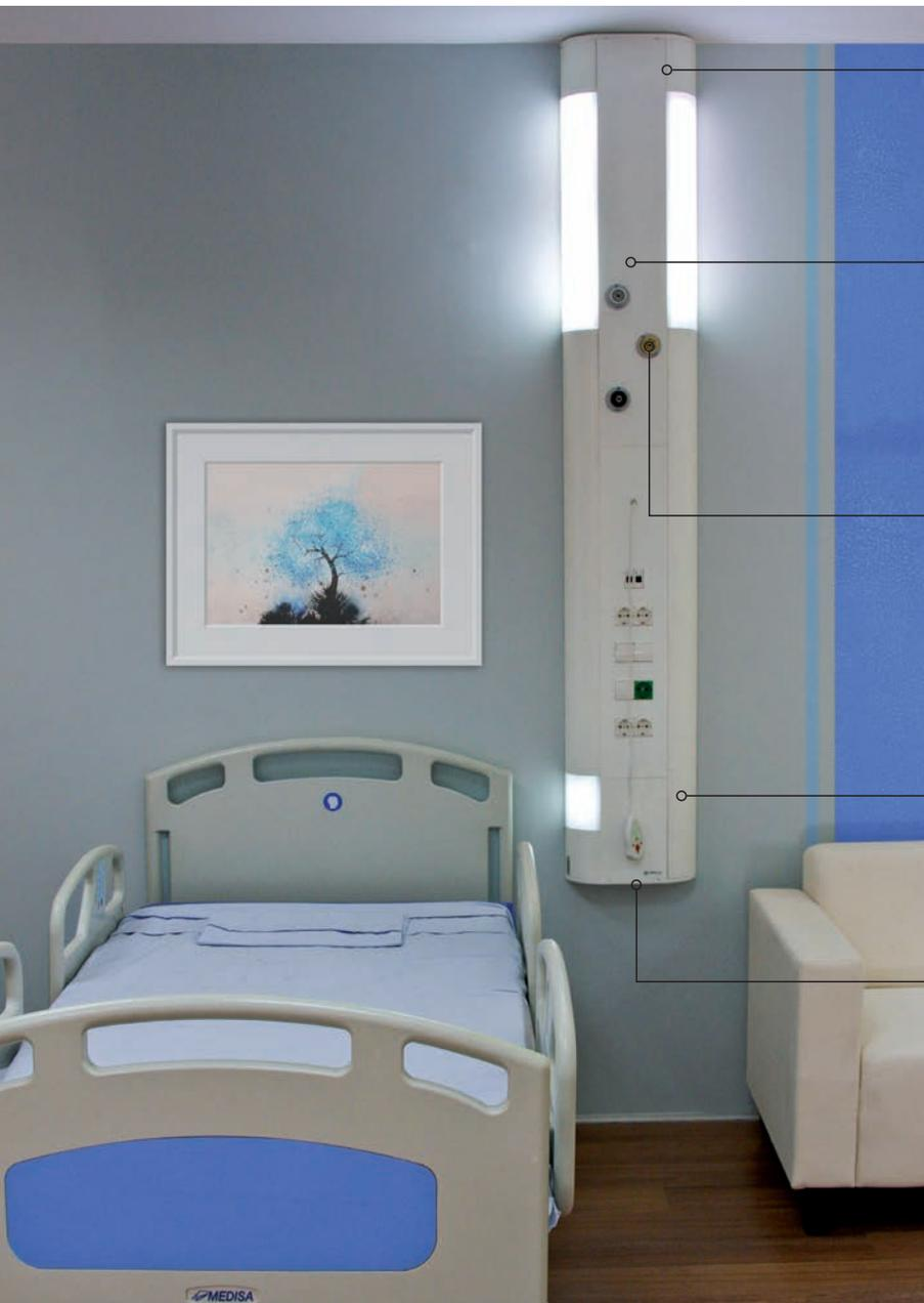
Access to inner parts of the Bed head unit is done by clipping system covers to avoid the visible screws.
